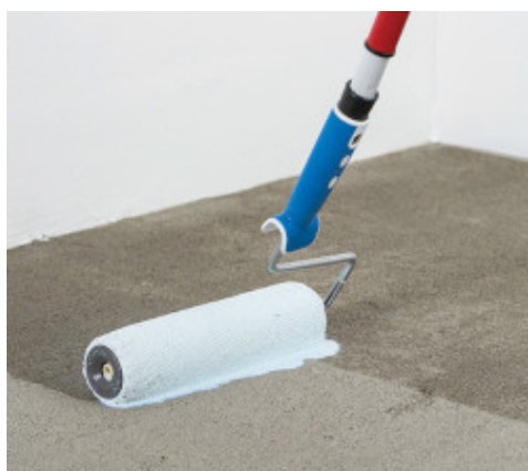
Primer application on the substrate
